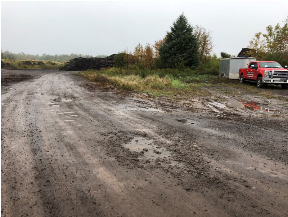
Area F2 Photo 1, Looking Northeast from Southwest:
