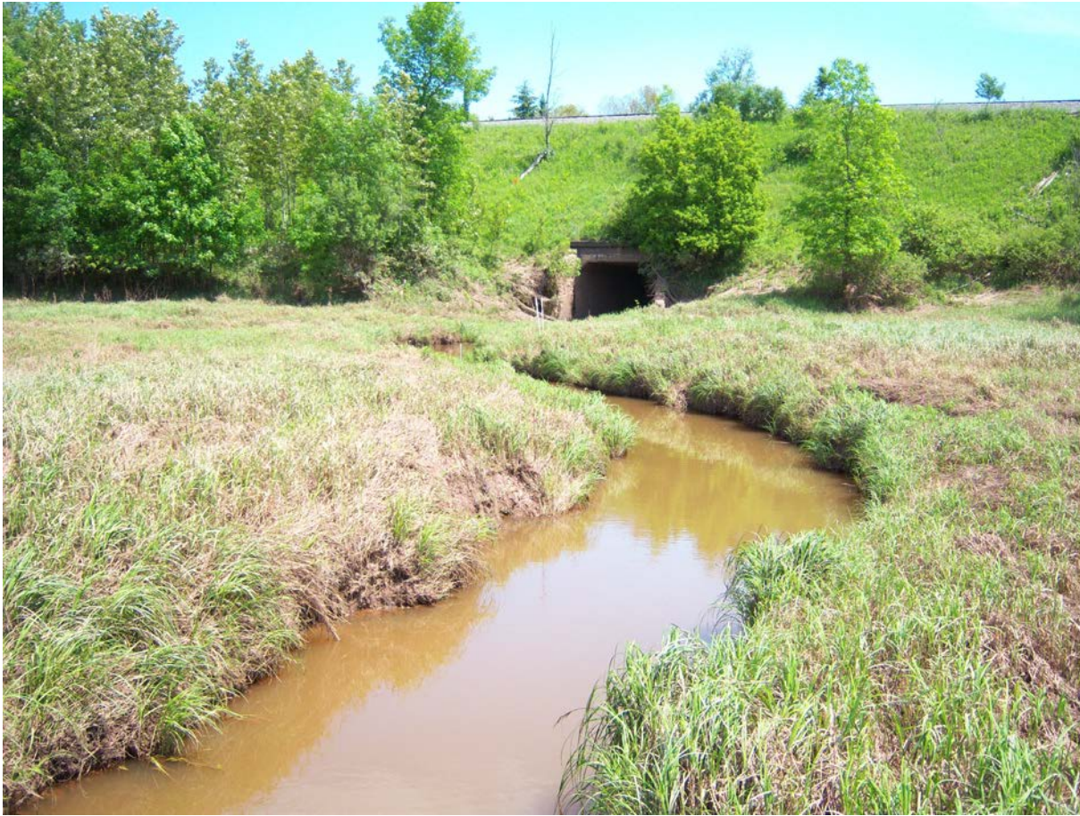
Crawford Creek and floodplain; looking NE (downstream) toward Soo Line RR Embankment and culvert
