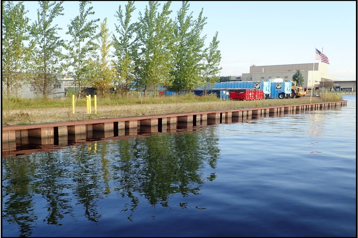
PHOTO 1. Overall view of the typical 2010 containment barrier wall, looking northwest.
