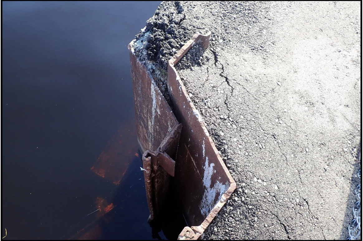
PHOTO 11. View of overlapping steel sheet piles at PT “E”.
