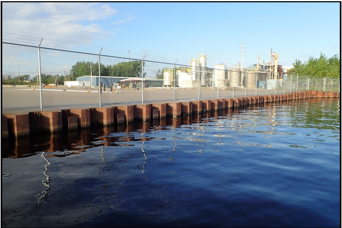
PHOTO 4. Overall view of the typical 1999/2000 containment barrier wall, looking southwest.
