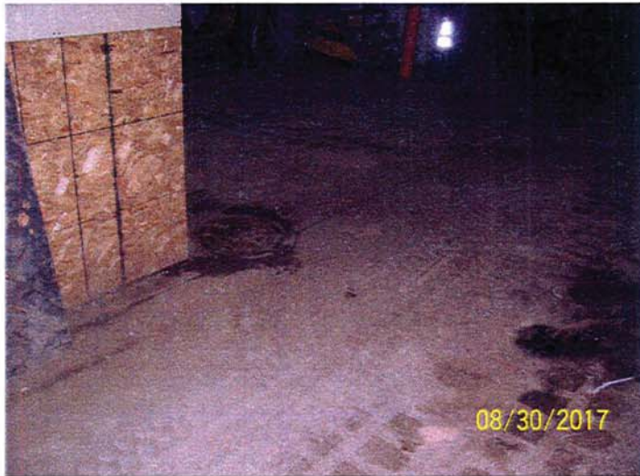
Title: Looking SW at W catch basin and concrete slab cap.
