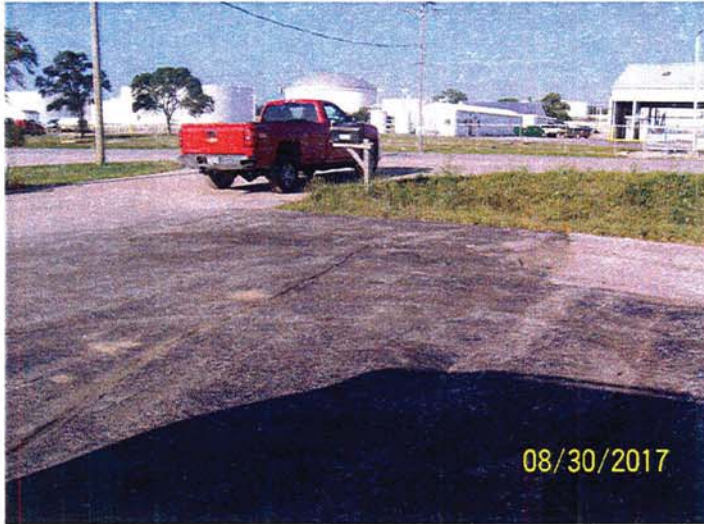
Title: Looking SW at asphalt parking area cap.
