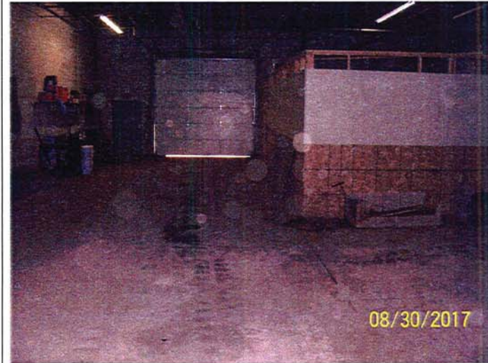
Title: Looking E at concrete slab cap.
