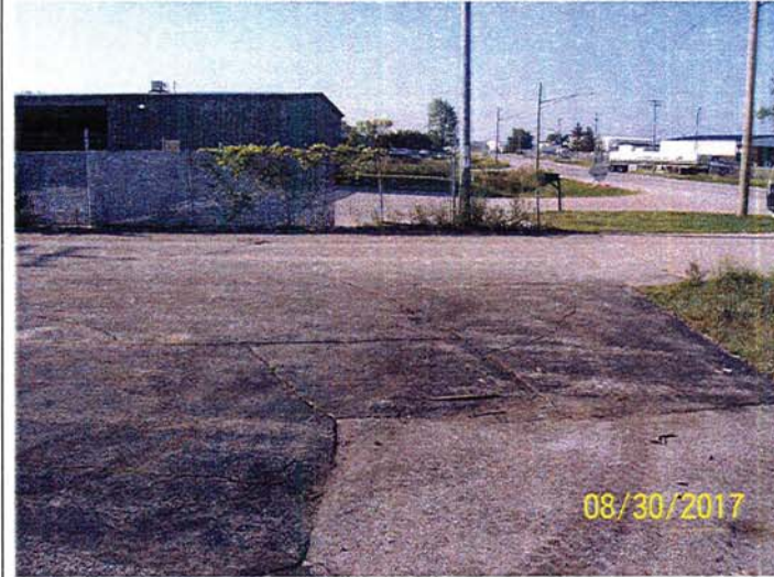
Title: Looking S at asphalt parking area cap.
