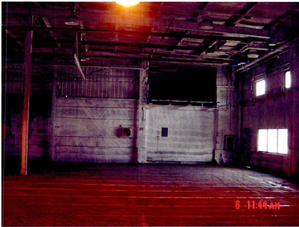
Former mercuric chloride mix room, northwestern corner of Building 7.
