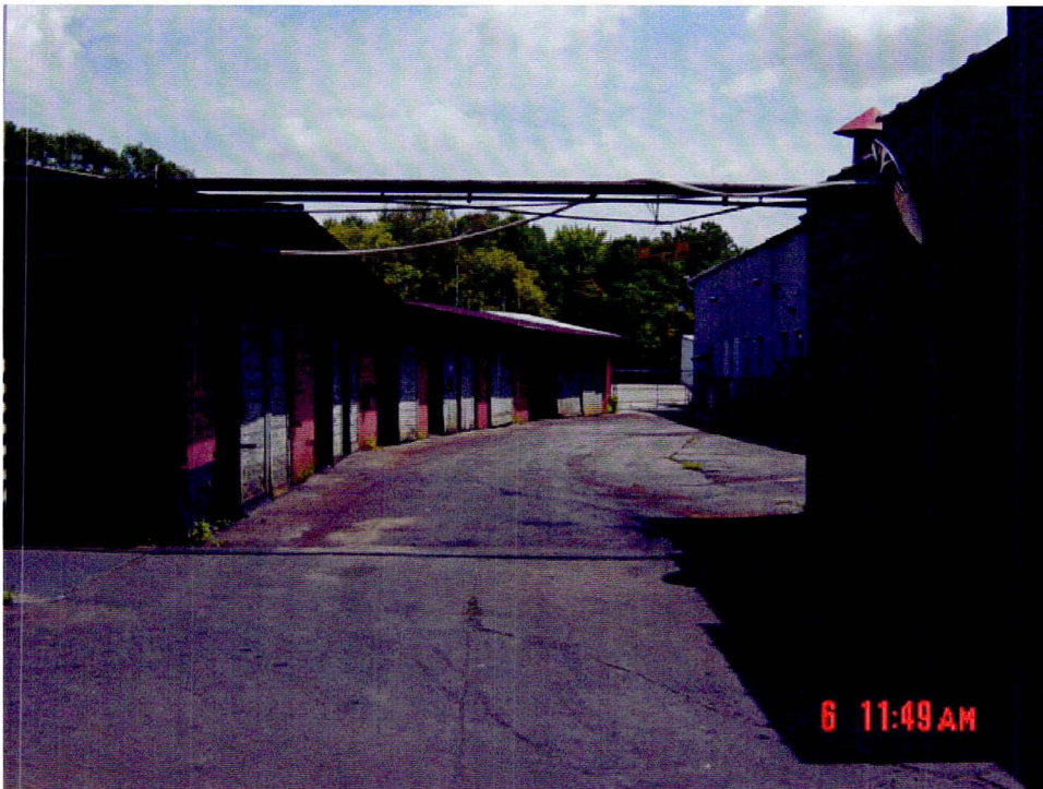
Buildings 23A, B, and C.
