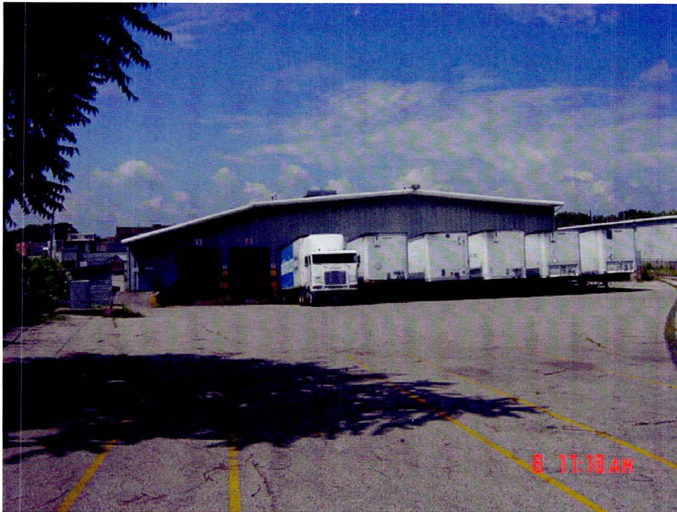
Looking at the eastern side of Building 11. This is also the location of site fill materials.
