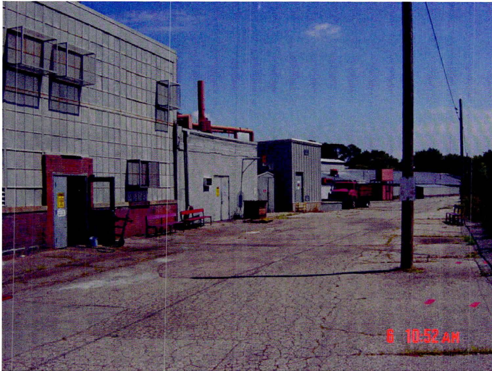
Location of former 10,000-gallon fuel oil UST, southern side of Building 5.
