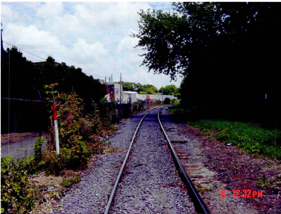
Railroad running parallel to the southern property border.
