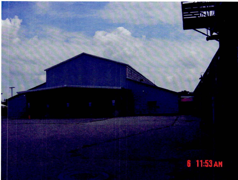
Western side of Building 15.
