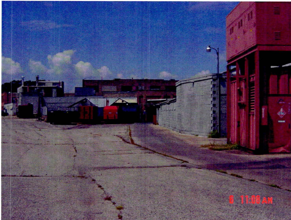
Location of two concrete holding USTs, southern side of Building 12C.
