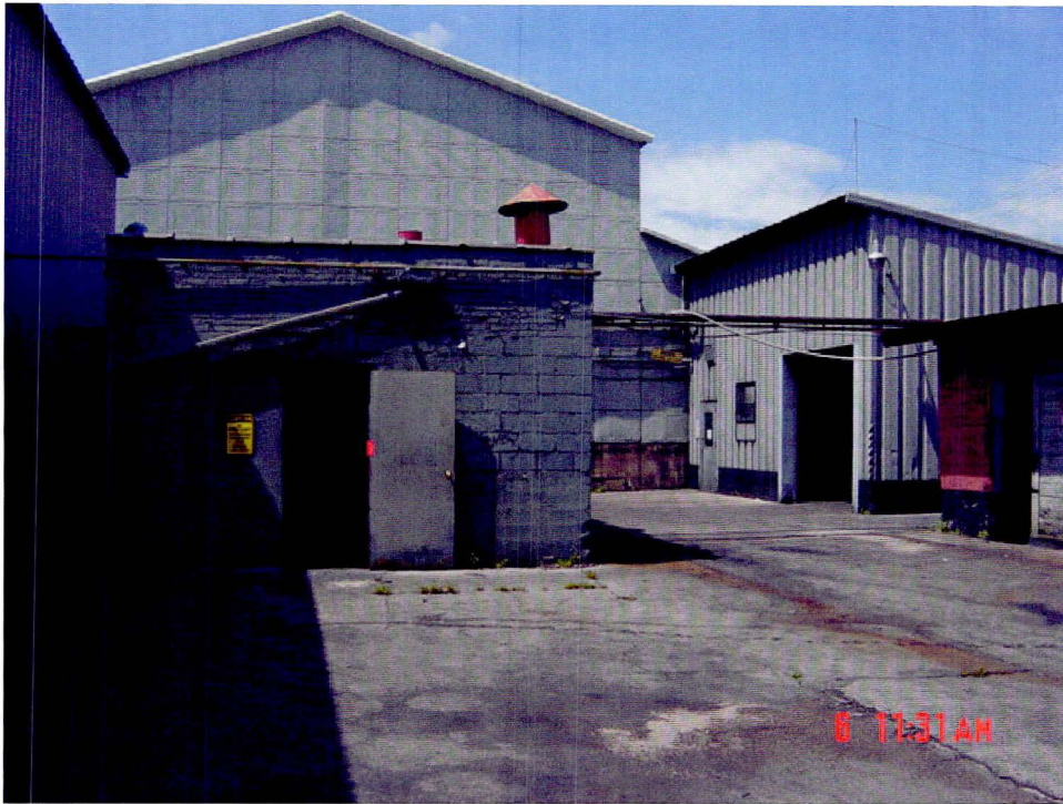
Compressor room number 2, Building 22.
