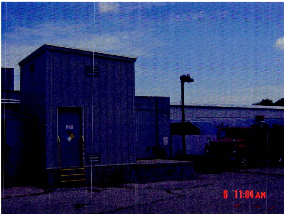
4,000-gallon fuel oil AST, southern side of Building 2.
