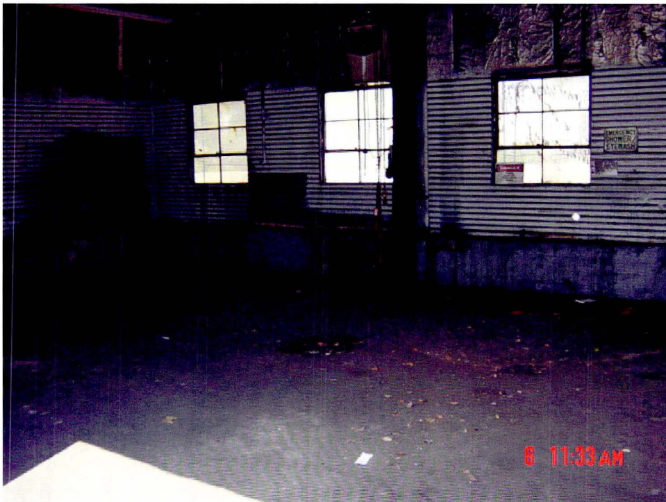
Truck garage, Building 10.
