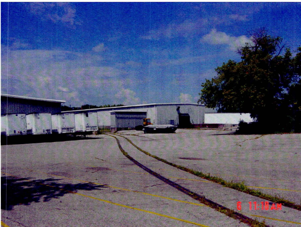
Looking at rail spur that enters the southeastern property corner and terminates by Building 7.
