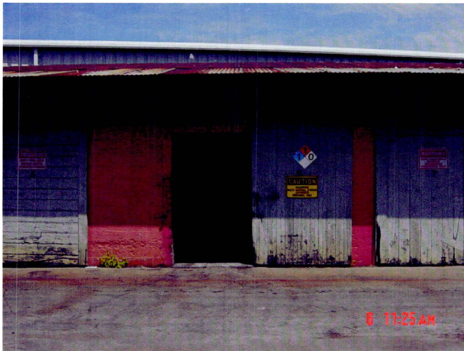
Hazardous waste accumulation area, Bin Number 6, Building 23B.
