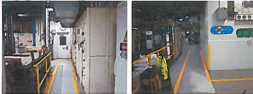
Exterior doorway/aisleway (exterior to CR-1)
