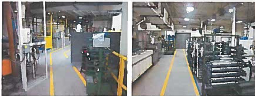
CR-1 (truss/roof supports) & electrical buss bars/plugs
