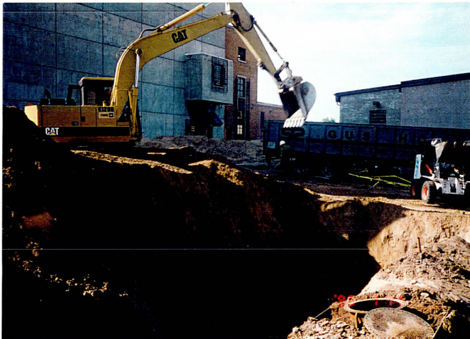
Photograph 4 July 14, 1995 Tank No. 1 area backfilled, Tank No. 2 being excavated.
