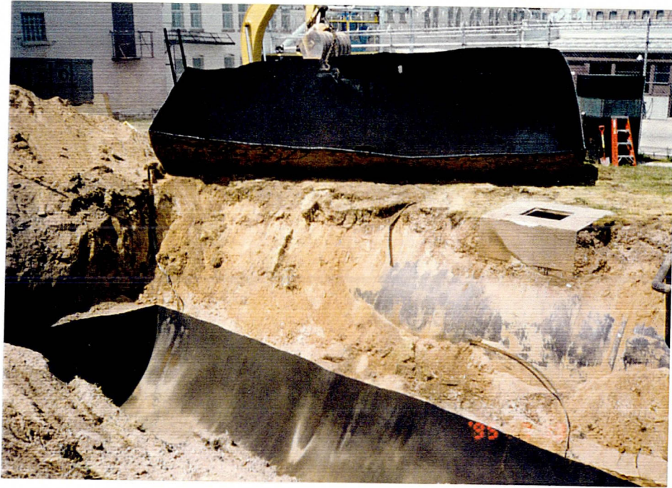
Photograph 3 July 13, 1995 Tank No. 1 cut and being removed from the excavation.
