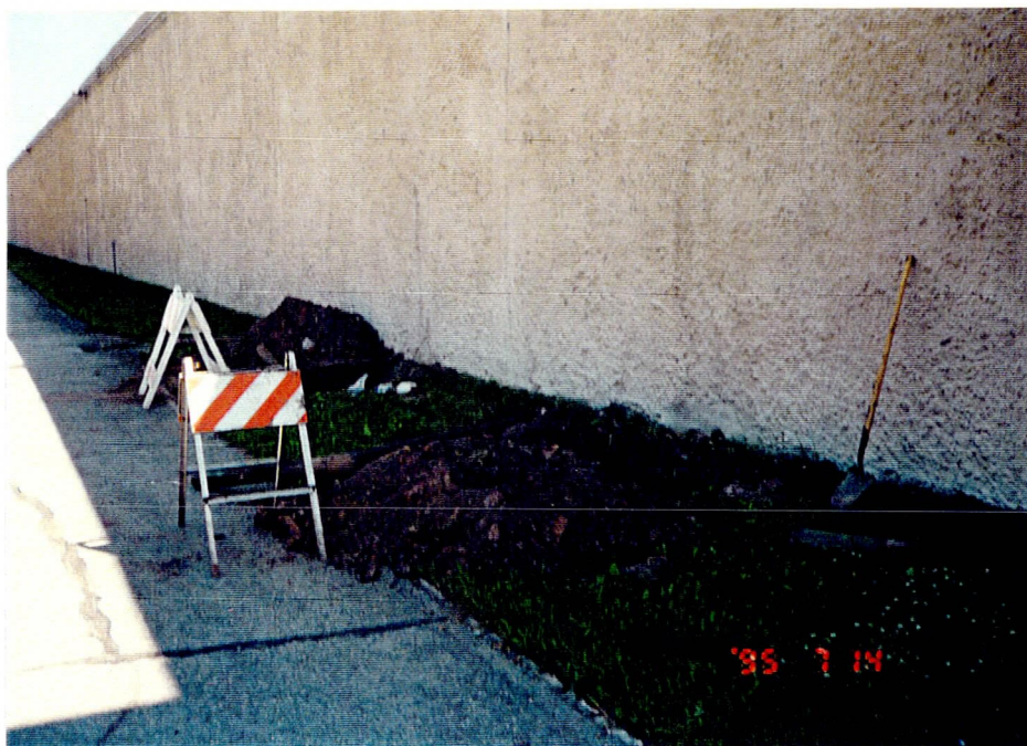
Photograph 8 Fill pipes outside of the prison wall, excavated, and removed.
