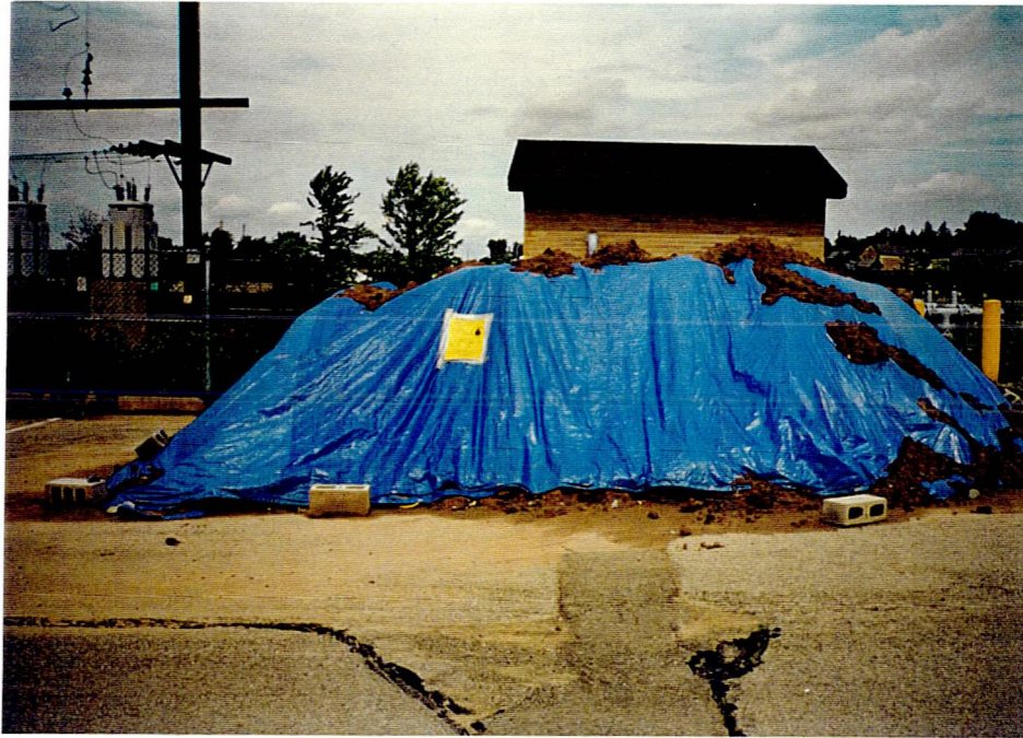
Photograph 9 August 3, 1995 Contaminated soil stockpile placed on paved parking lot, covered with a tarp, and displaying warning sign.
