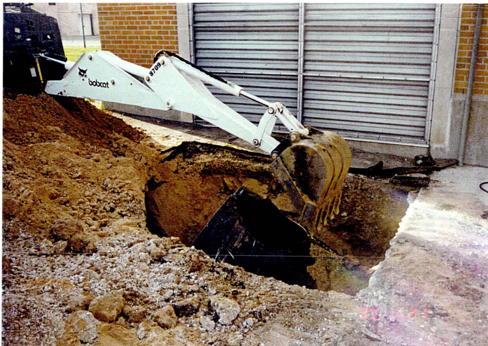
Photograph 10 November 21, 1995 1,000-gallon diesel tank being removed.
