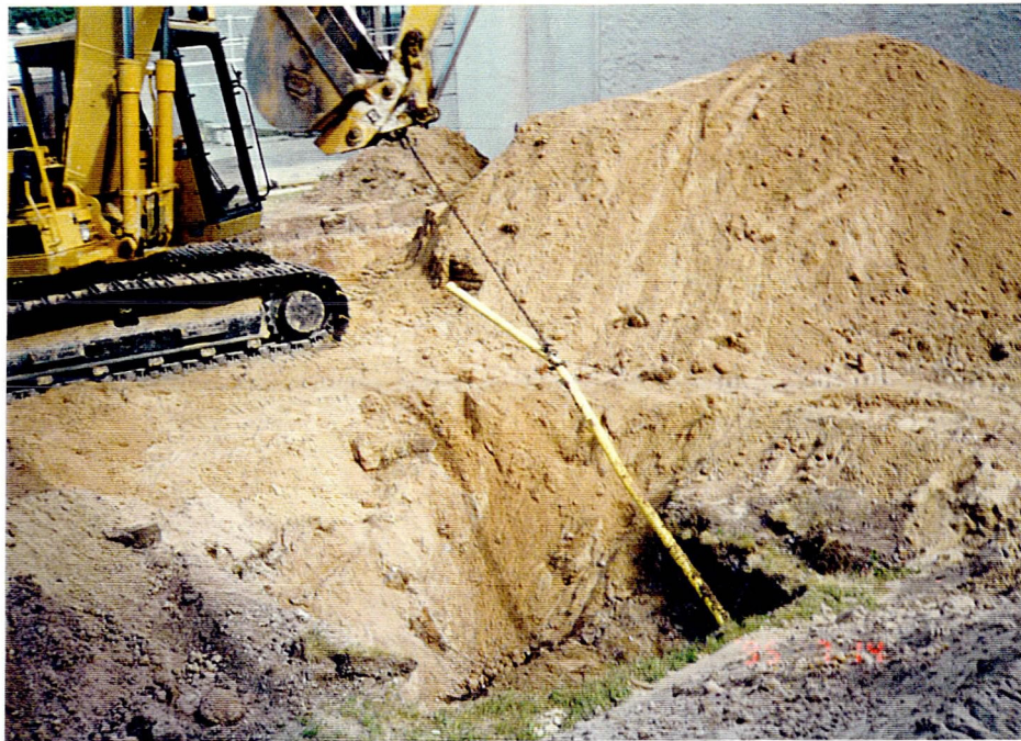
Photograph 7 Fuel lines being removed.
