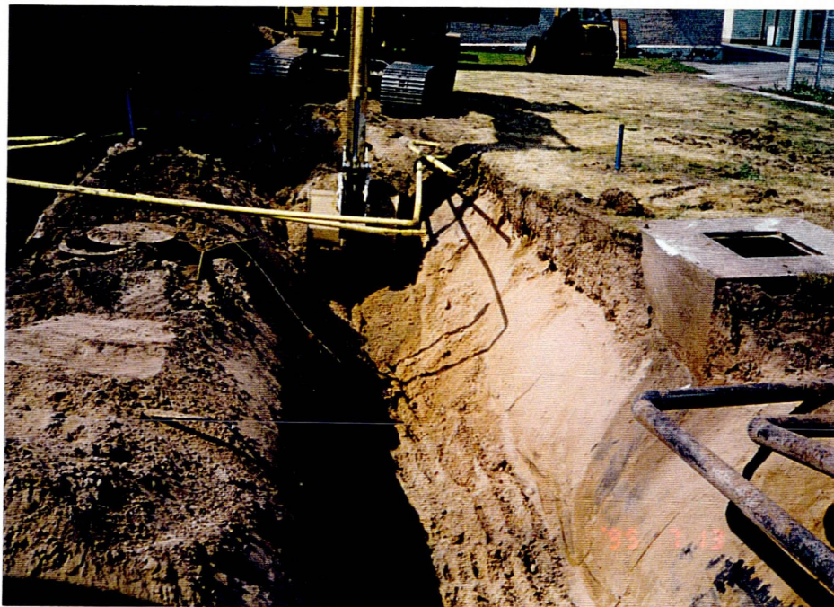
Photograph 2 July 13, 1995 Excavating Tanks No. 1 (east tank, on left) and No. 2 (west tank, on right).
