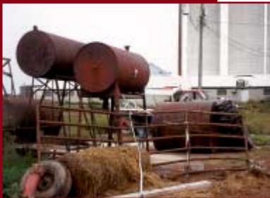
2. Check your storage tank's stability. A typical 250 gallon tank supports a ton of fuel oil when full. This necessitates a strong and stable supporting structure. Have your tank's base inspected at least once a year. Storage tanks located on steep grades or exposed to harsh weather conditions are especially vulnerable. The second photo on the left details an unreliable support structure. Note the fallen oil tank next to the supports.
