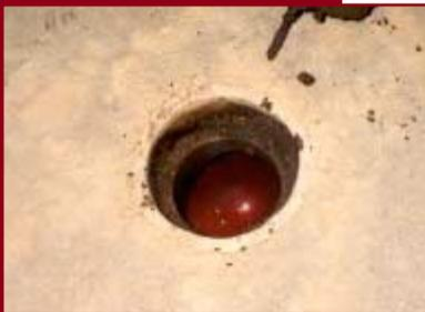
6. To prevent overfills, you should ensure that the fuel oil level gauge is functioning properly and accurately. Specify the quantity of fuel needed to the supply company and request that your tank's size and existing quantity of fuel in the tank is verified before fueling. The last photo on the left shows fuel oil in a basement floor opening resulting from an overfill.
