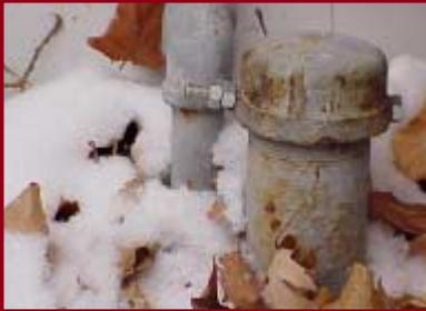
1. If you have a disconnected fill pipe that leads into your basement, you should cancel service with your fuel oil company immediately. In addition, remove the fill pipe or secure the cap with a bolt to make accidental filling more difficult (see first photo on the left). Clearly mark any pipelines still in service for easy recognition.
