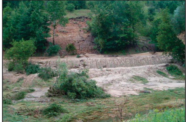
Figure 12: Landslide from August 2007 flood in Coon Creek Watershed.
