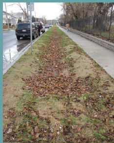
Urban BMPs can be used to generate credits for WQT.
