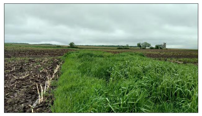
Figure 6: Photo of existing grassed waterway facing upslope at Site Photo Location #3 (see Figure 1)
