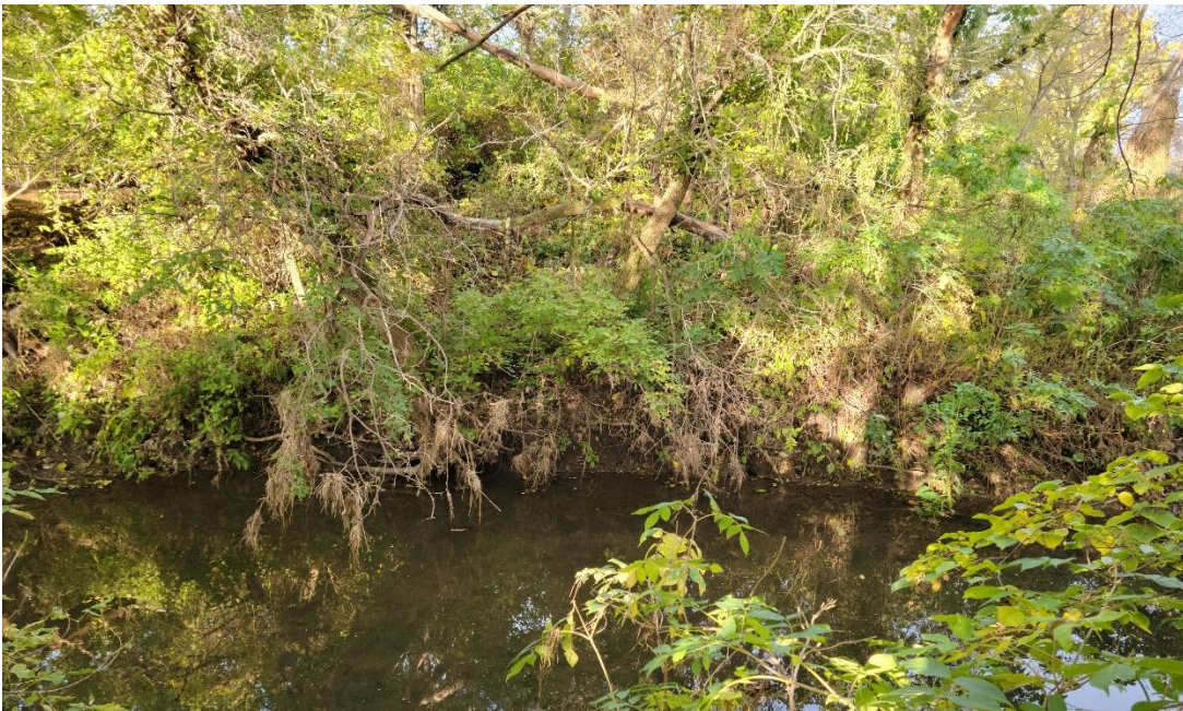
Severe undercut with vegetative overhang and exposed tree roots.
