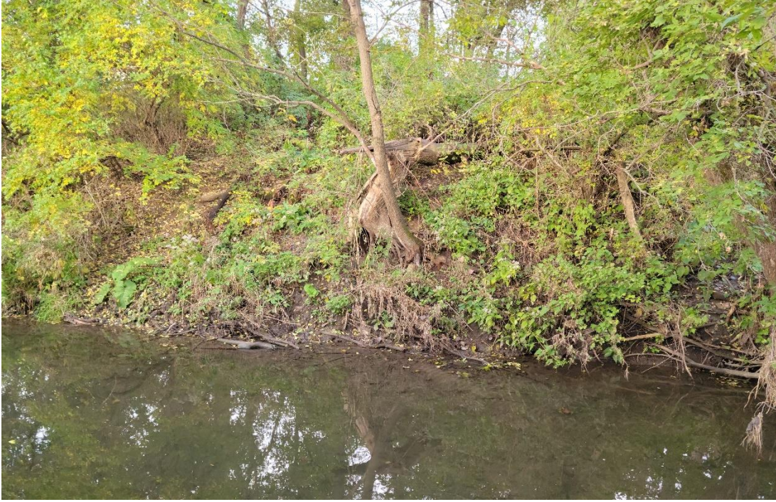
Severe undercut with vegetative overhang and exposed tree roots.
