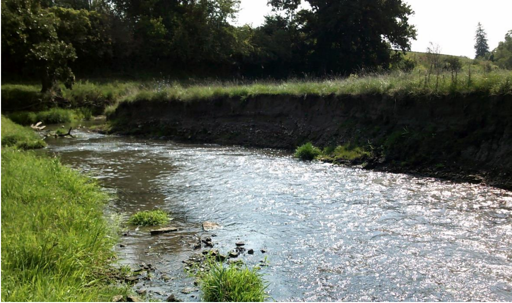
Image 8 – Bare bank, severe undercut with slump and vegetative overhang.
