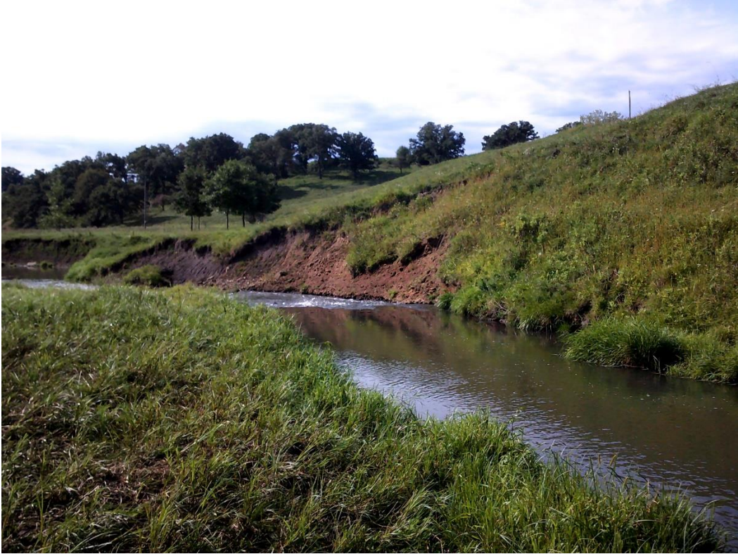
Image 13 – Bare bank, severe undercut with slump and vegetative overhang.
