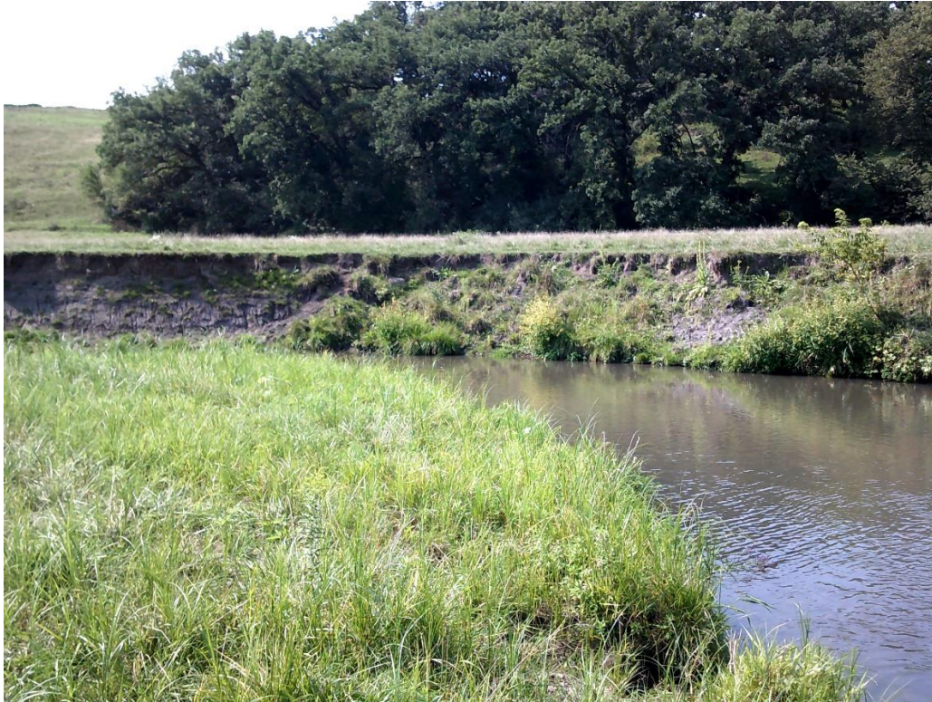
Image 6 – Bare bank, severe undercut with slump and vegetative overhang.
