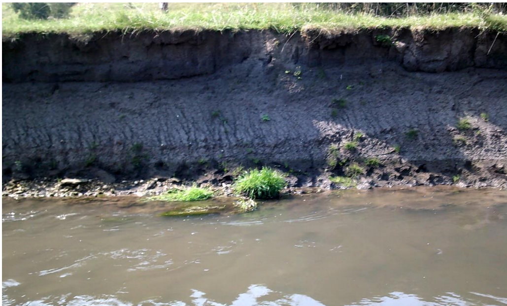
Image 7 – Bare bank, severe undercut with rills, slump, and vegetative overhang.
