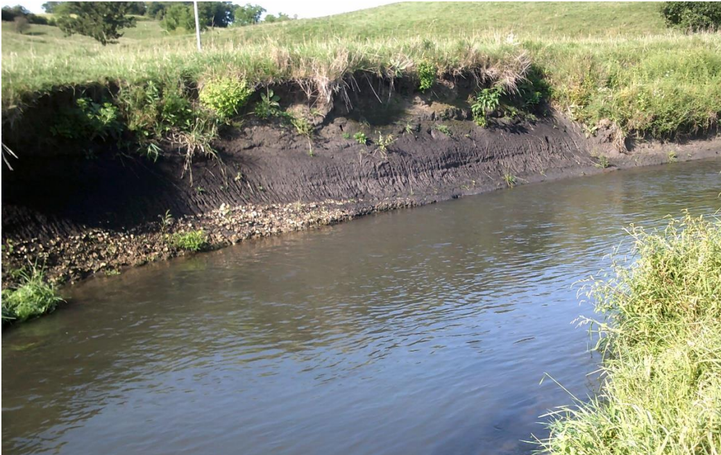
Image 11 – Bare bank, severe undercut with rills, slump, and vegetative overhang.
