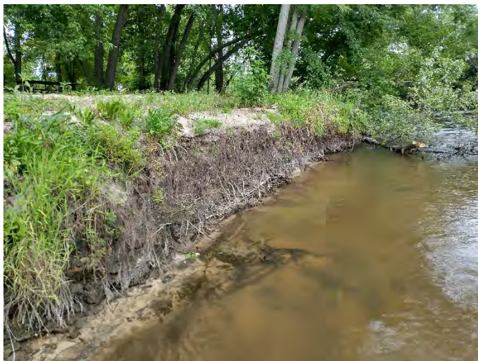
5: Bank erosion, north side of river
