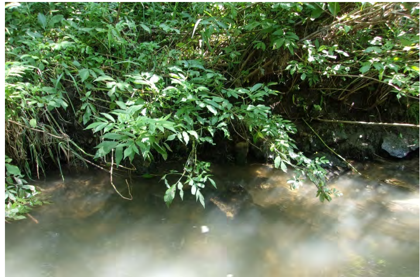
3: Closeup of undercutting on Bruce Valley Creek
