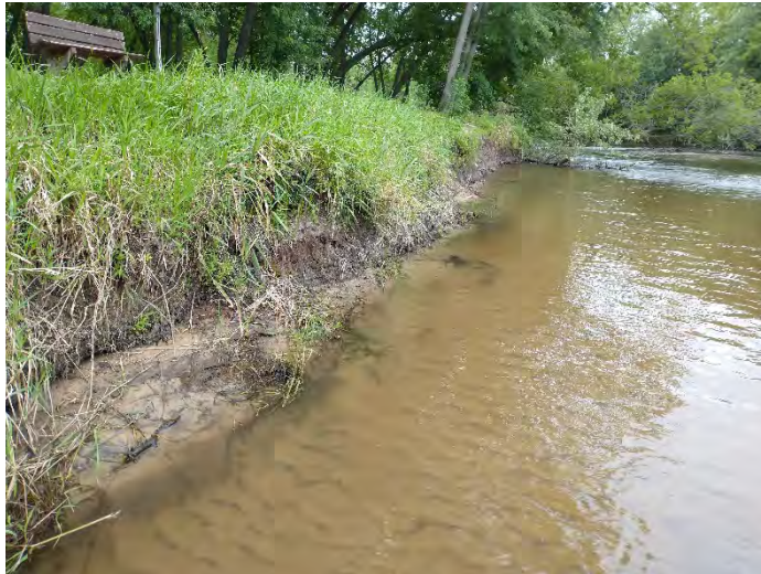
3: Toe cutting and erosion, north bank
