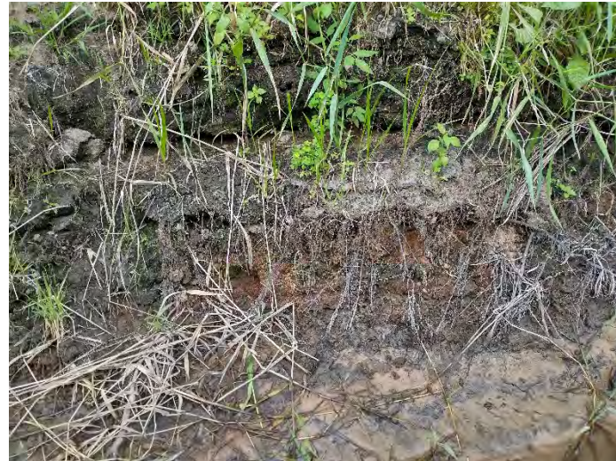
4: Toe cutting and erosion, north bank
