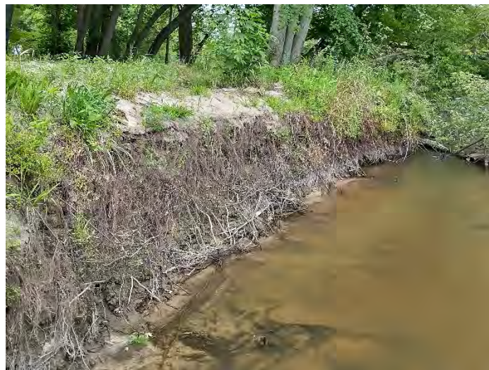
6: Bank erosion, north side of river
