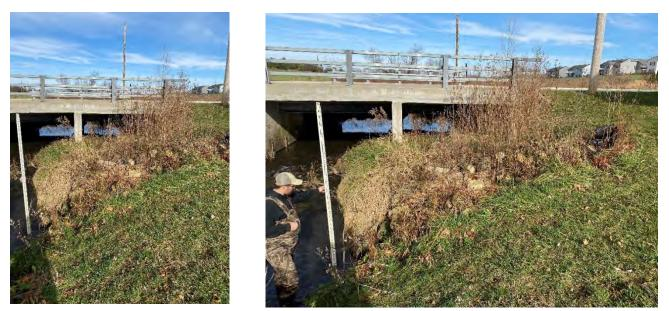
Figure 46.0: Sta. 57+35-57+75 Slight. Vegetative overhang and outfall exposed.
