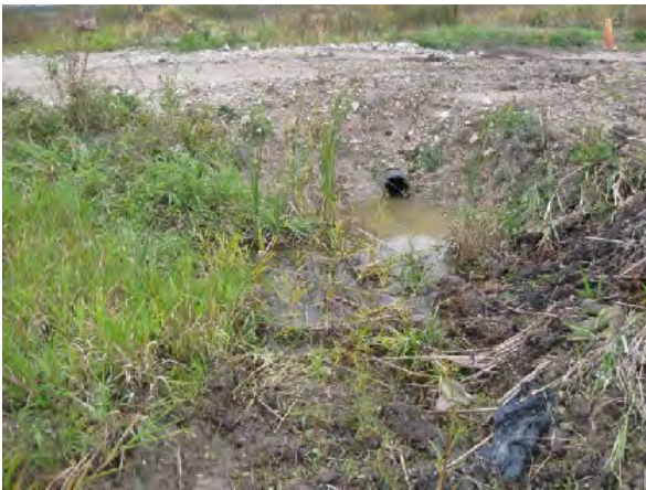
W3 and culvert connection to W2, view Northwest
