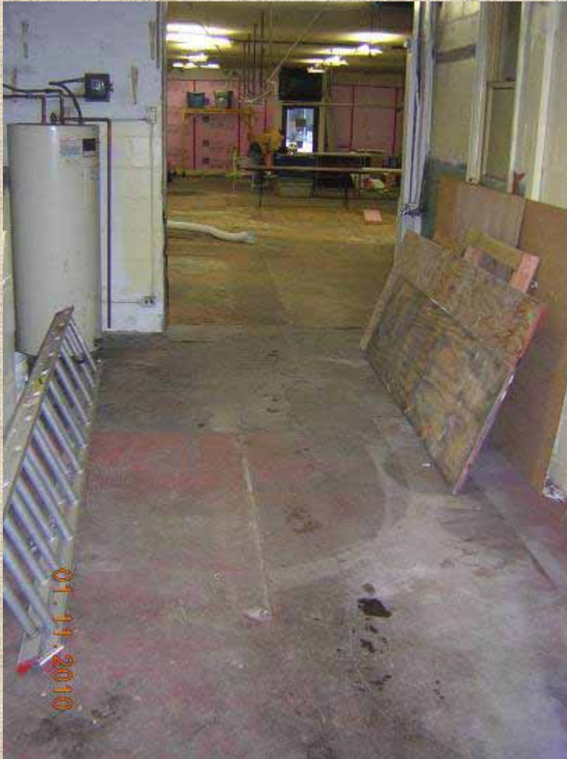
Looking south towards store front area
