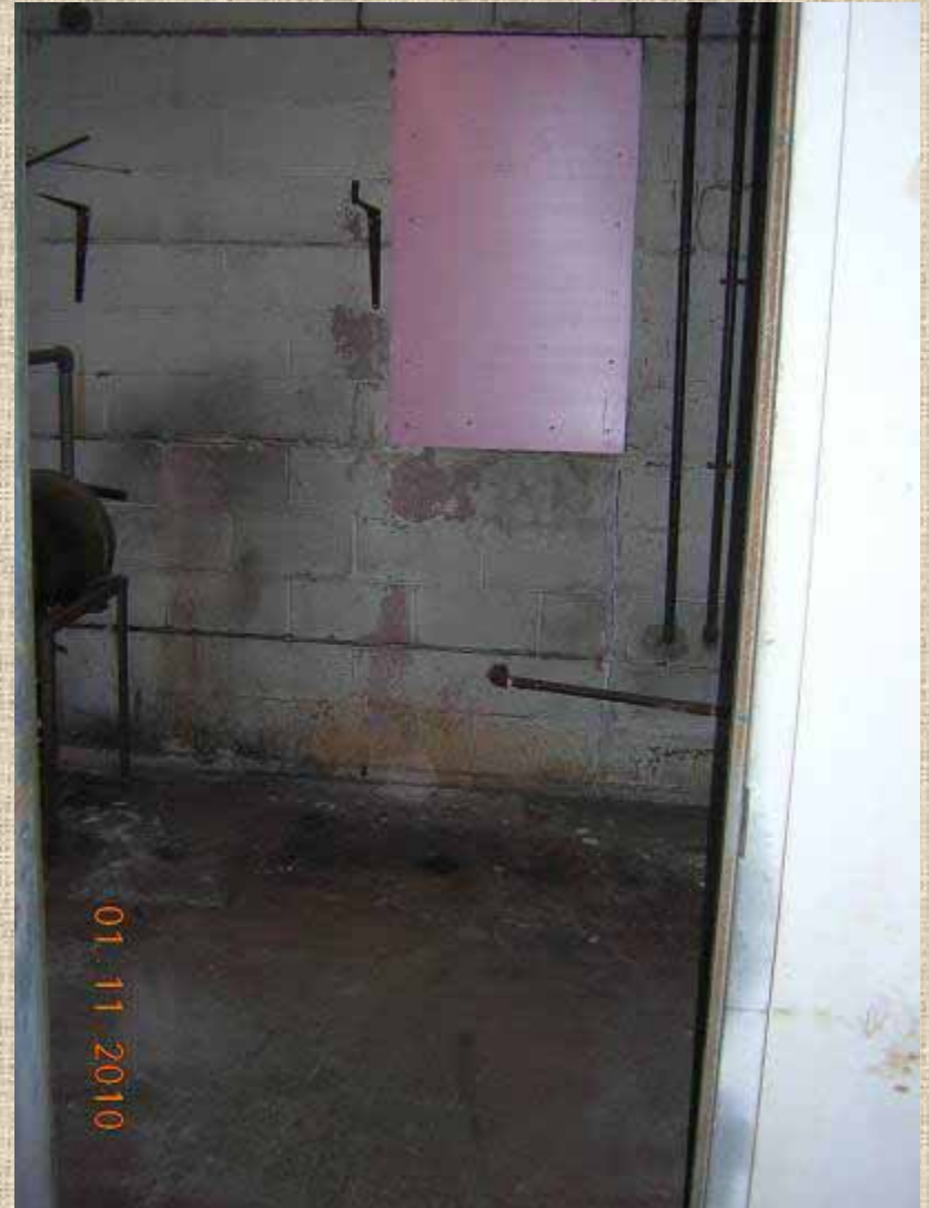
Looking north into boiler room
