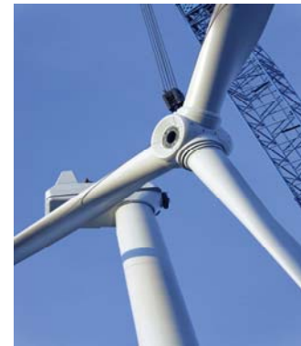
MGE Wind Farm
