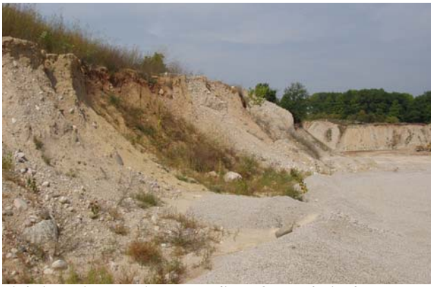
Kiel site prior to primary grading of gravel pit slope, August 2005.
