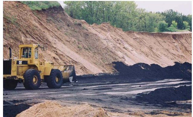
Foundry sand used as fill needed to achieve favorable post-mining contours during mine reclamation at the Foley Pit. (Photo by Tom Portle)
