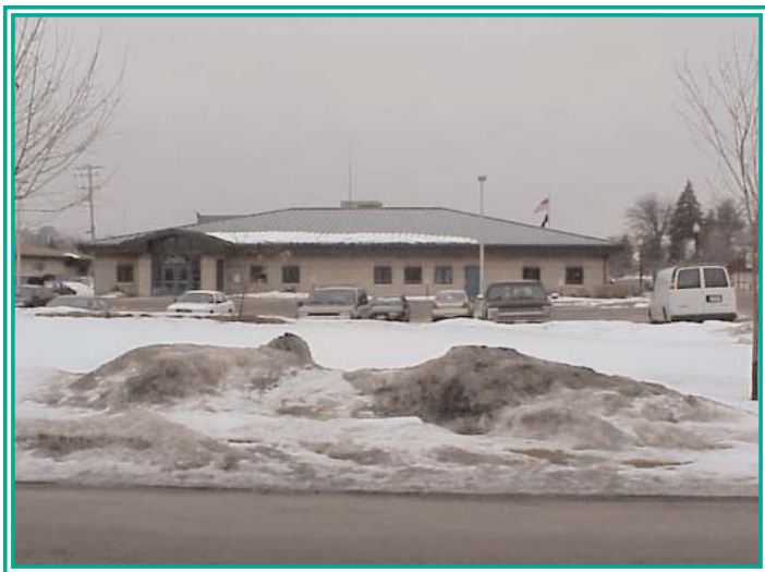
The DeForest Public Safety Building after redevelopment was complete (DNR photo).
