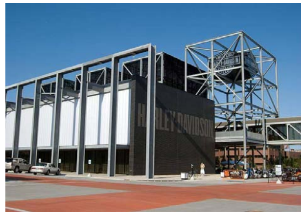
The Harley Museum in Milwaukee's Menomonee River Valley, built on four former brownfield properties (DNR photo).
