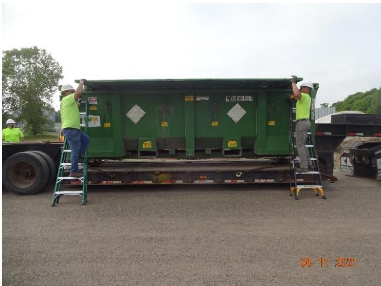
7. View of steel lid being closed on loaded roll off box.
