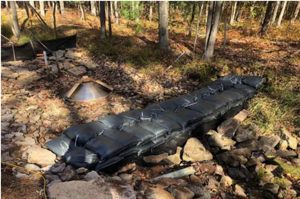
Photograph 2. Ditch A In-stream check dam after maintenance completion.
