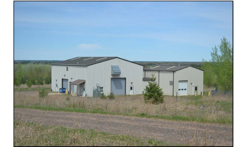
TREATMENT BUILDING AT PENTA WOOD PRODUCTS SITE
