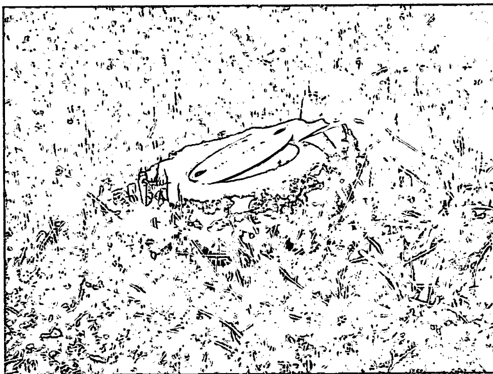
Figure 6 Monitoring well MW116 at Chrome Shop not sealed properly (winter heaving or settling problem).
