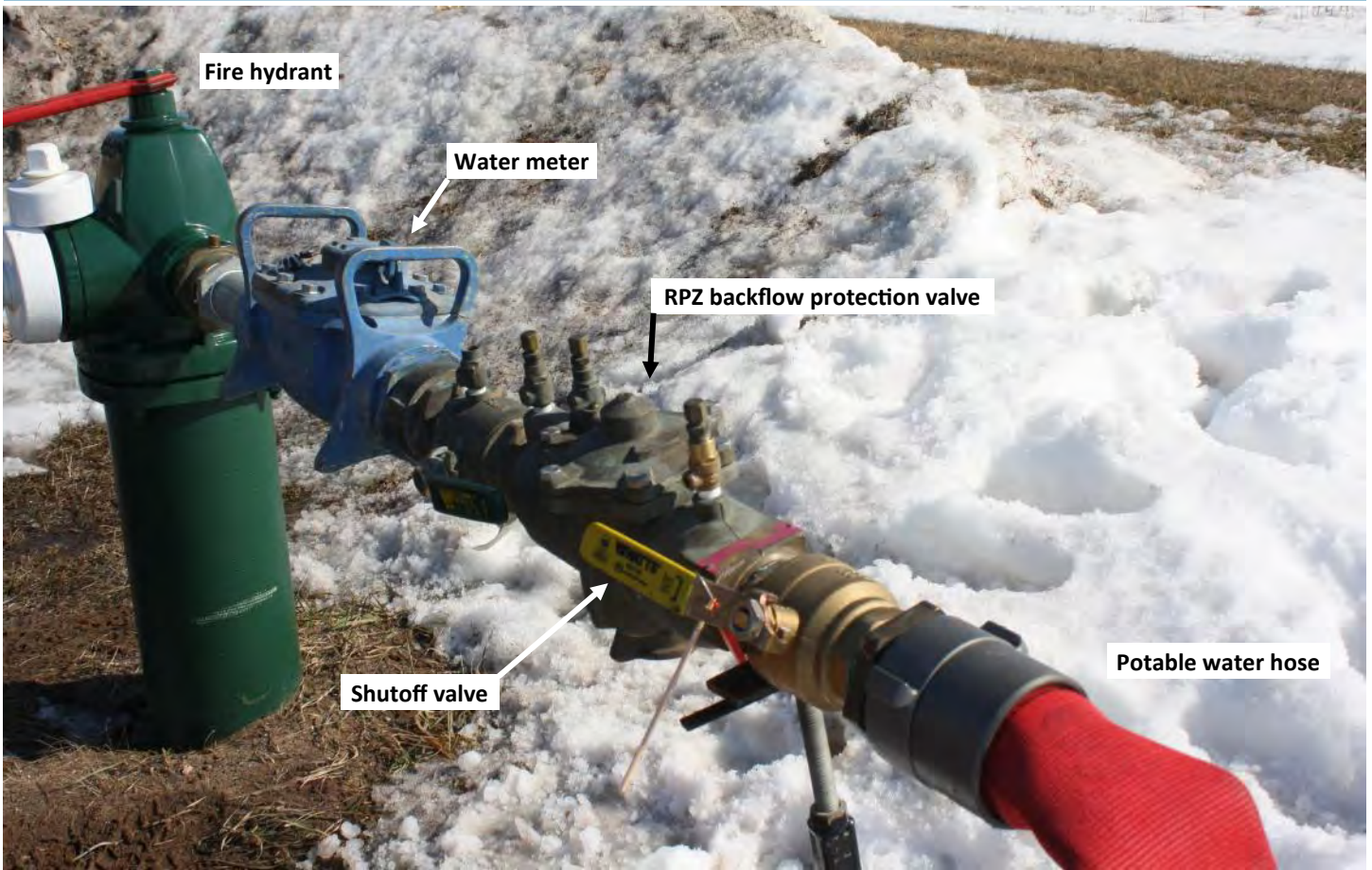
Use the correct materials and hook up your temporary water supply properly, and you will be prepared to deliver safe drinking water throughout your event!
